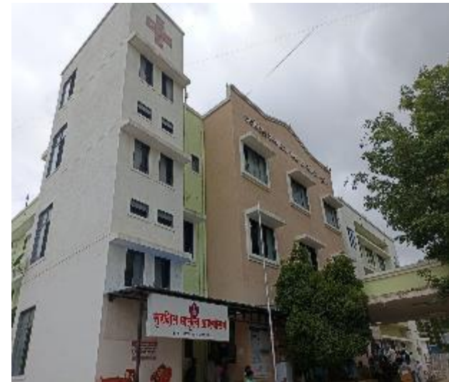
Image 1: Sub district hospital, Manchar
