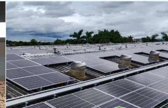
Transition to Solar renewable power (2.6 MW current installed capacity)
